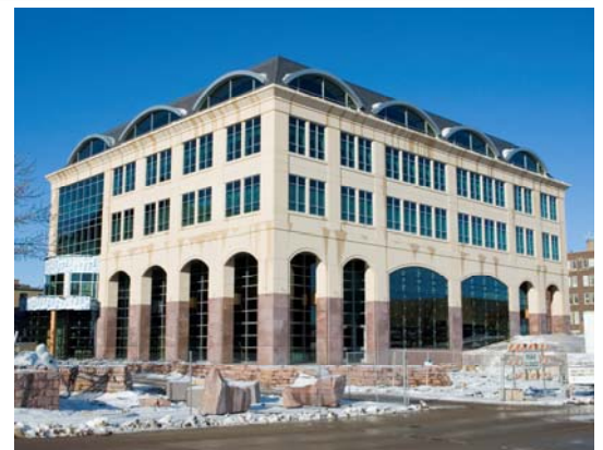
Courthouse Square under construction
