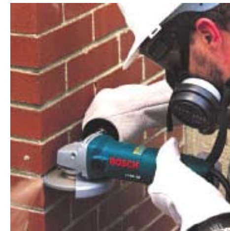
Cutting out old mortar.
