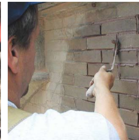
Applying new mortar.
